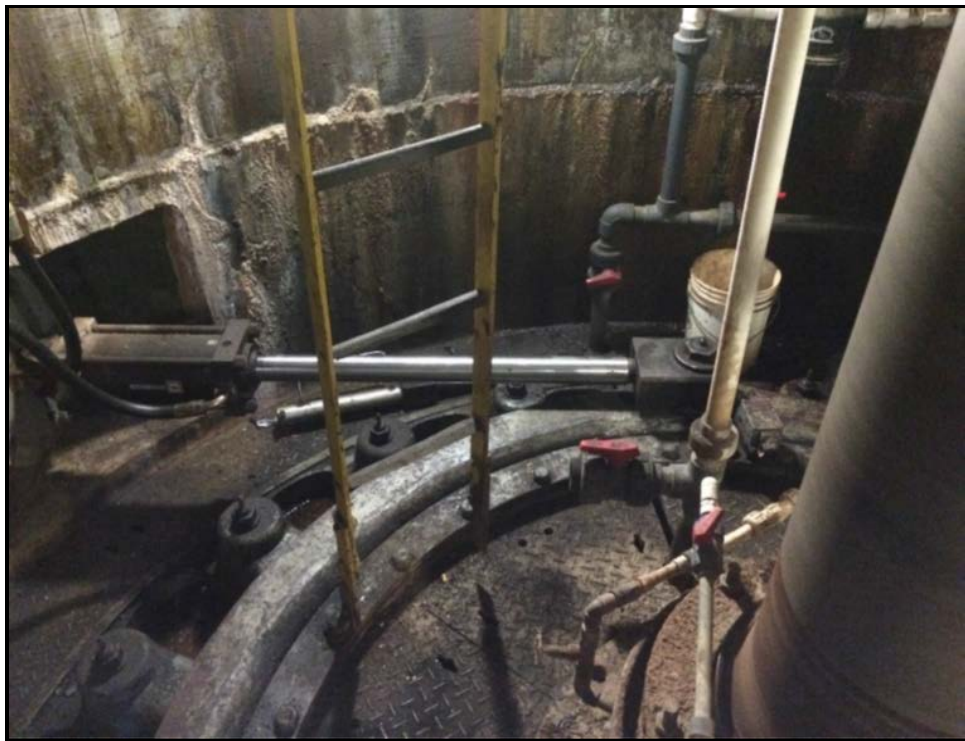
PHOTO 4-1 PARR SHOALS DAM PIPING FOR VACUUM BREAKERS IN HEADCOVER
